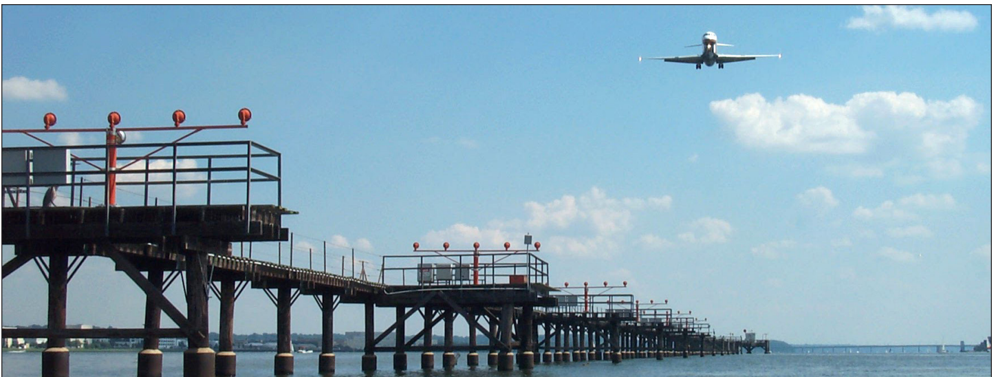
Runway approach lighting at Runway 1 at Ronald Reagan Washington National Airport. At 2,094 meters in length Runway 1 has an approach lighting structure out into the water to a distance of 820 meters from the threshold.
