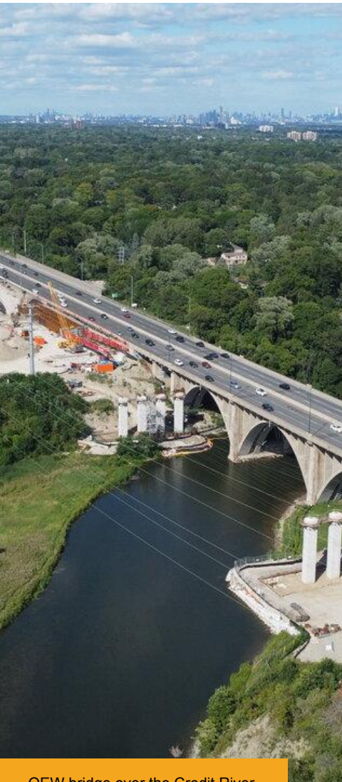
QEW bridge over the Credit River
