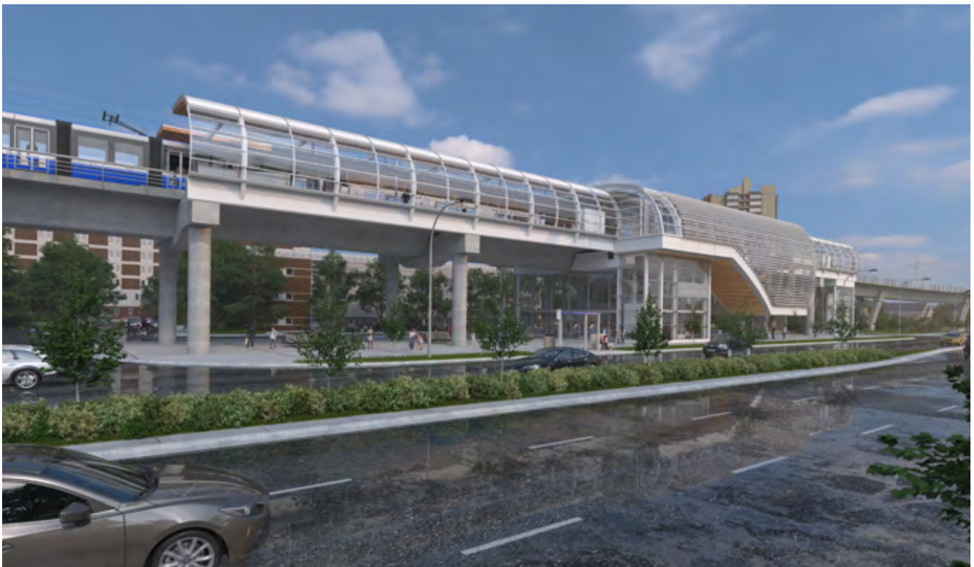
Artist Rendering of the Misericordia Transit Station, Valley Line LRT Photo credit: City of Edmonton
