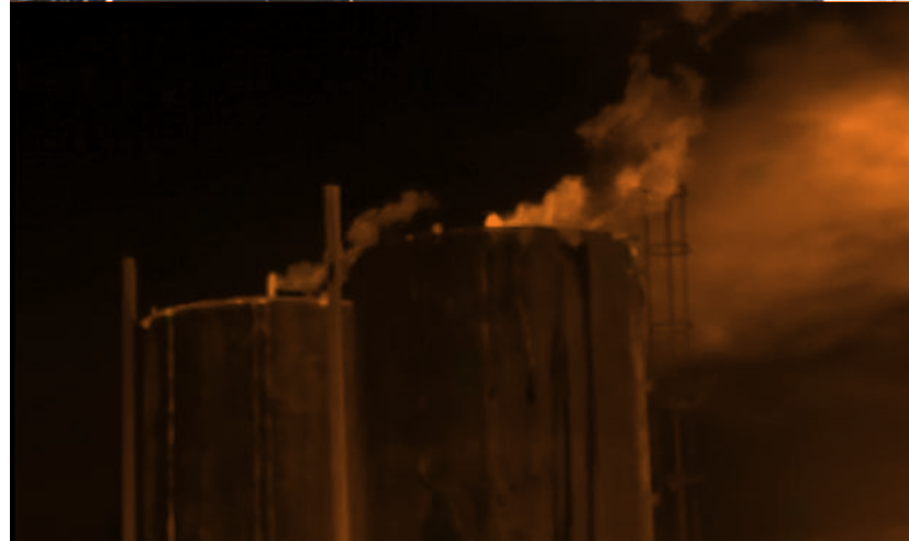
INFRARED CAMERAS REVEAL WHAT THE NAKED EYE CAN'T SEE: CONSTANT METHANE LEAKS FROM HEAVY OIL TANKS
